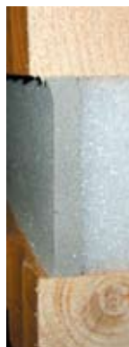
Replace plastic liner over the surface of the sealant
