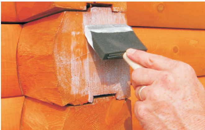
Applying Log End Seal
